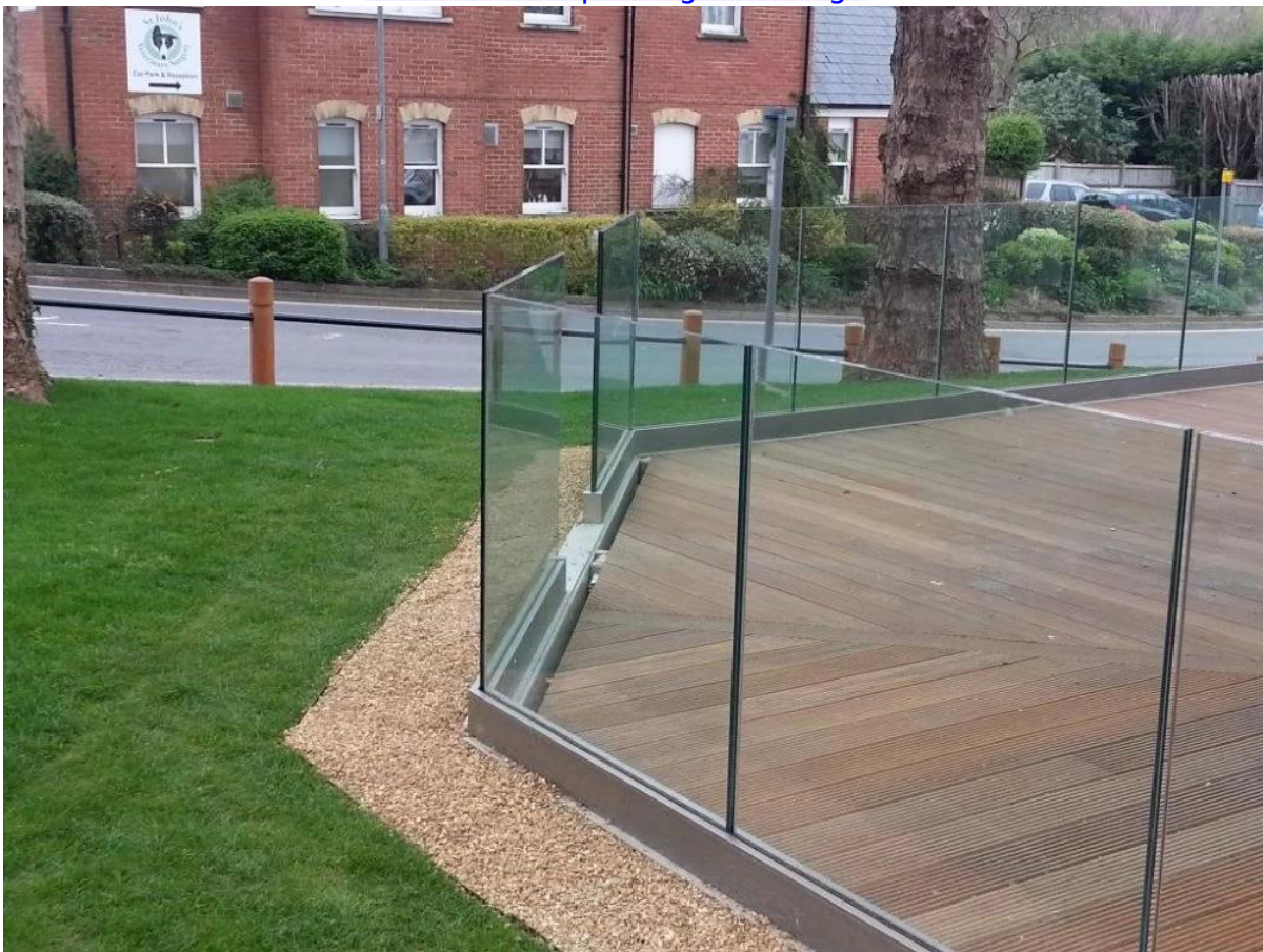
Aluminum U channel + 10-12mm tempered glass design
