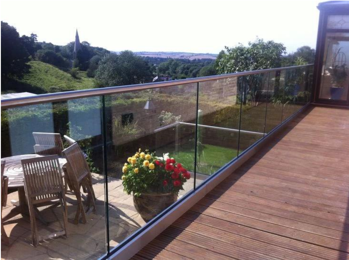
Aluminum U channel + 10-12mm tempered glass design
