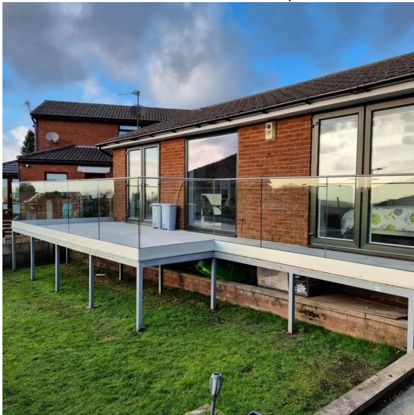
Base Aluminum U channel with Round stainless steel top rail
