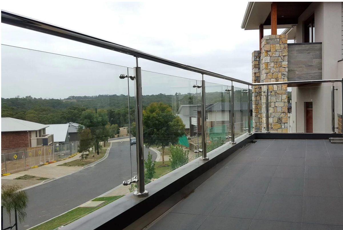
Spider glass fittings handrail project photos
