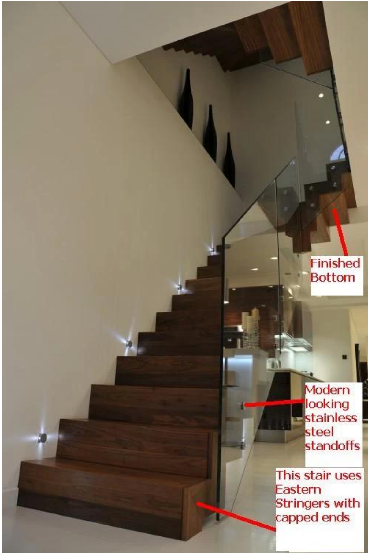
More project photos for glass rail standoff after installation :
