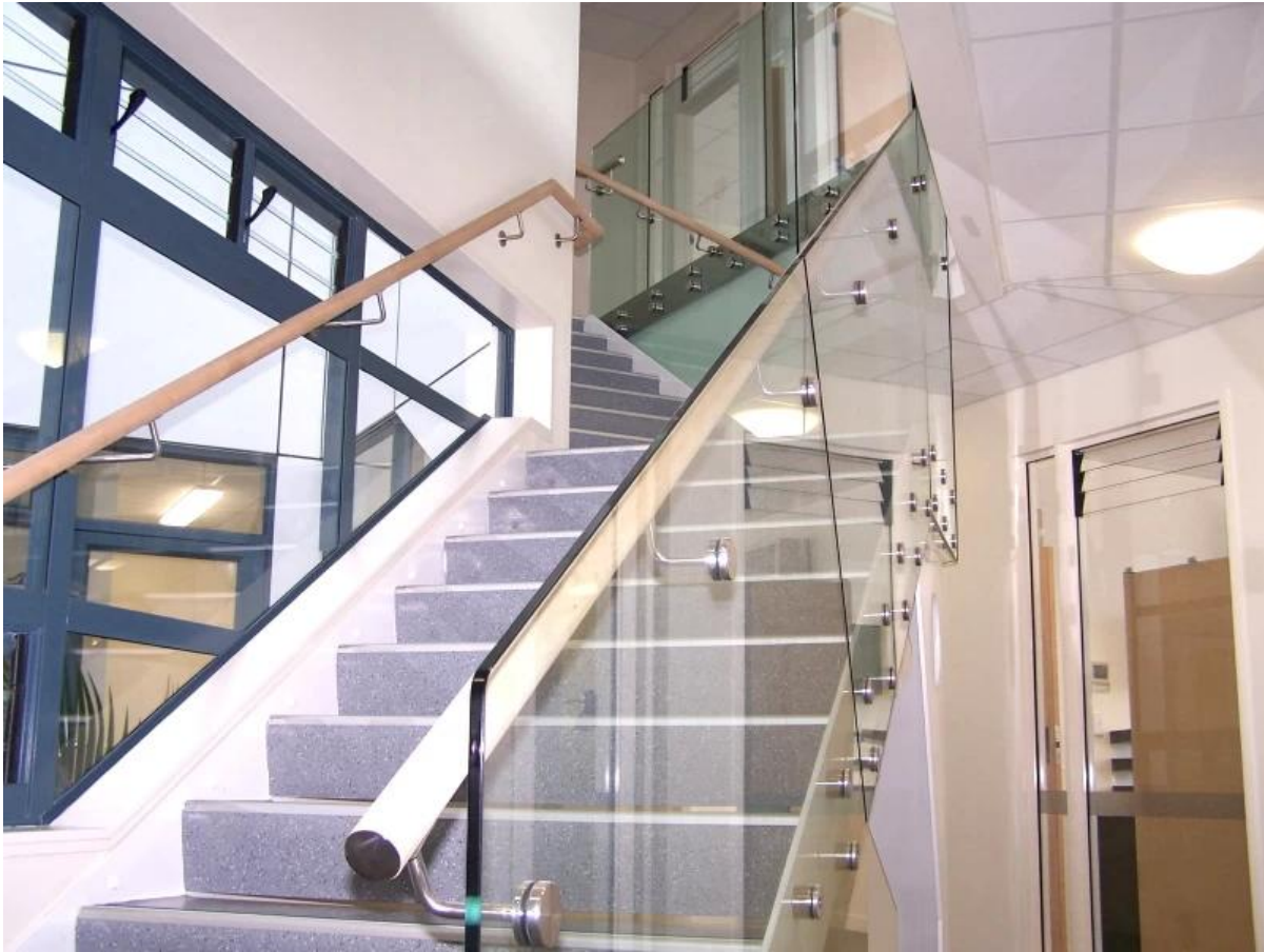
(2) Glass spigot railing design
