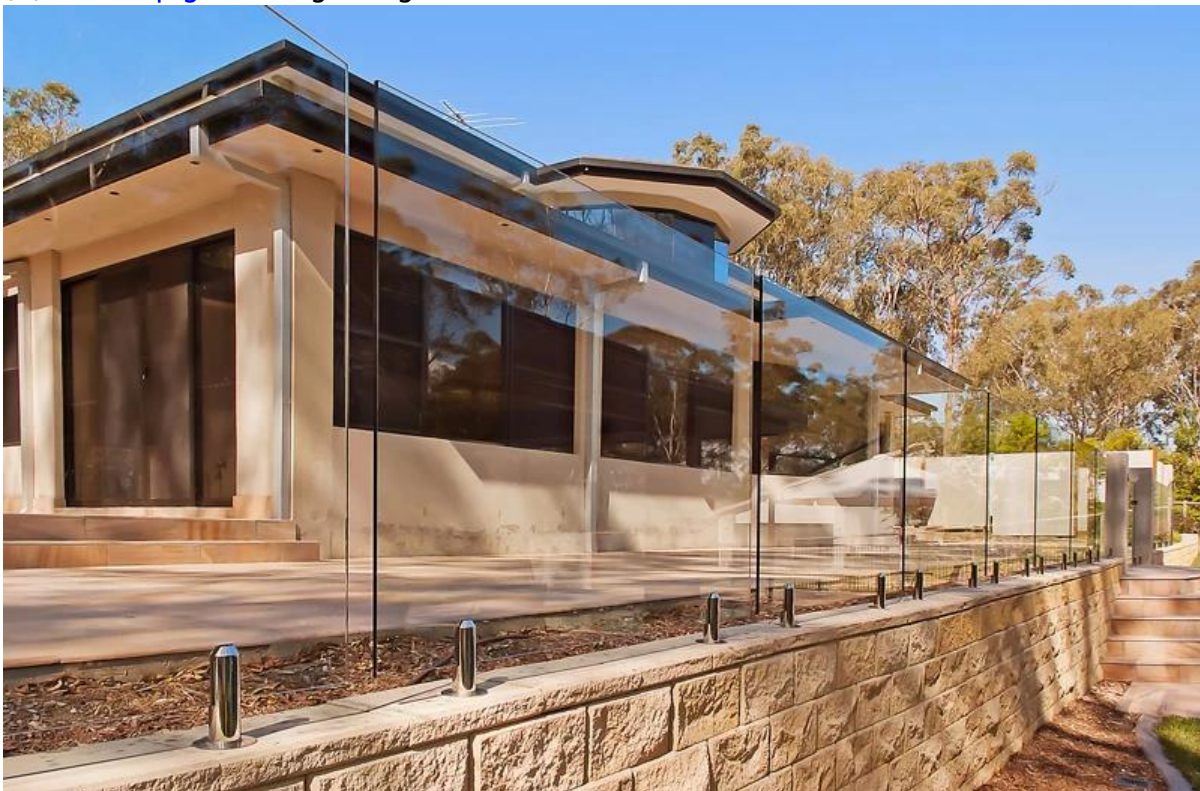
(2) Glass spigot railing design
