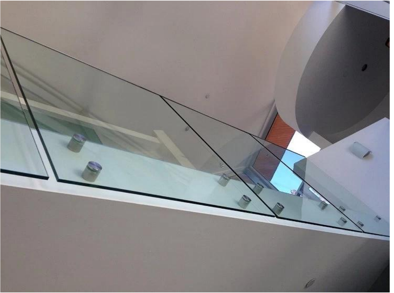
stainless steel standoff bracket for glass railing design
