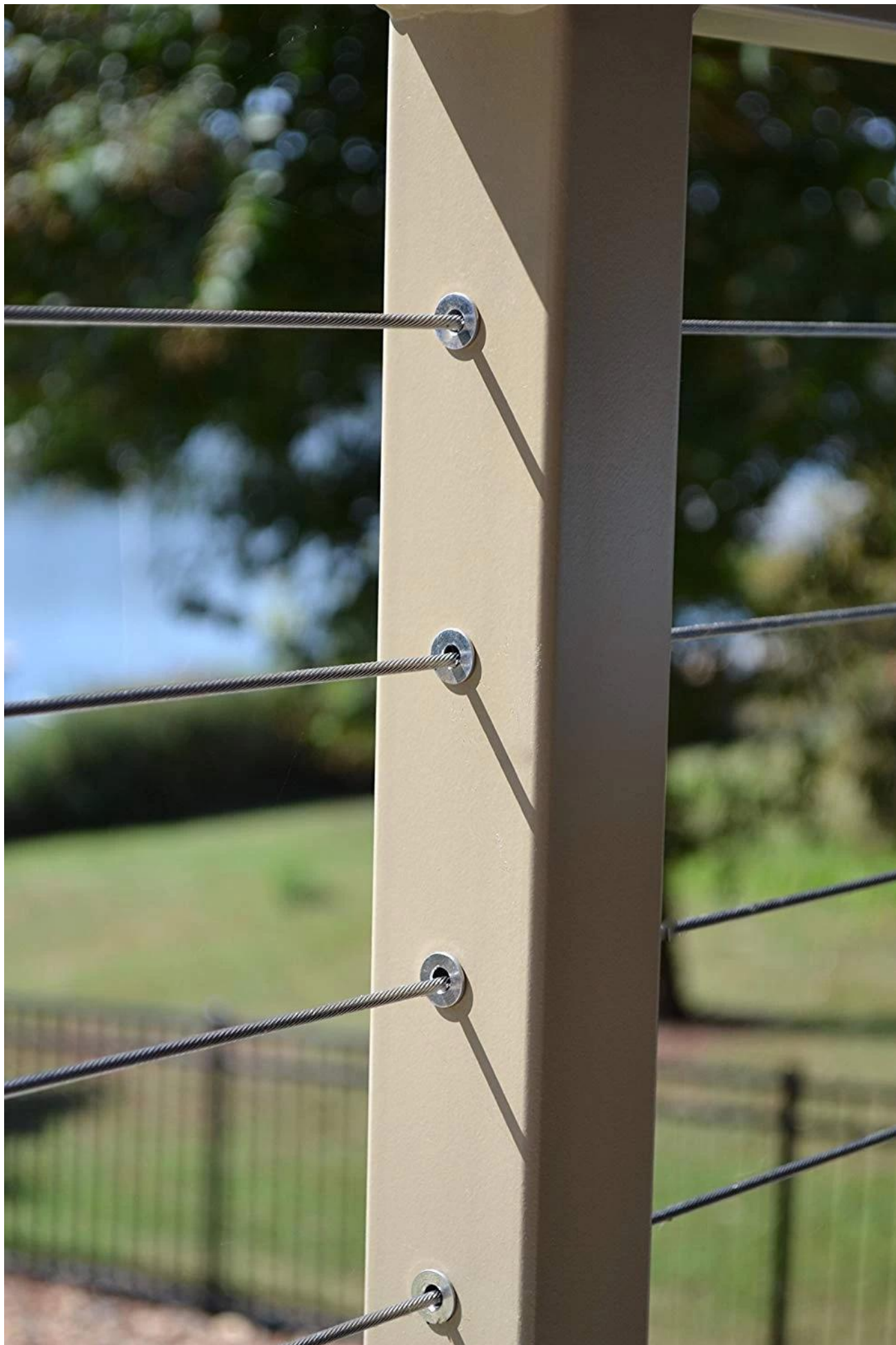
Type 316 stainless steel has the best corrosion resistance among standard stainless
