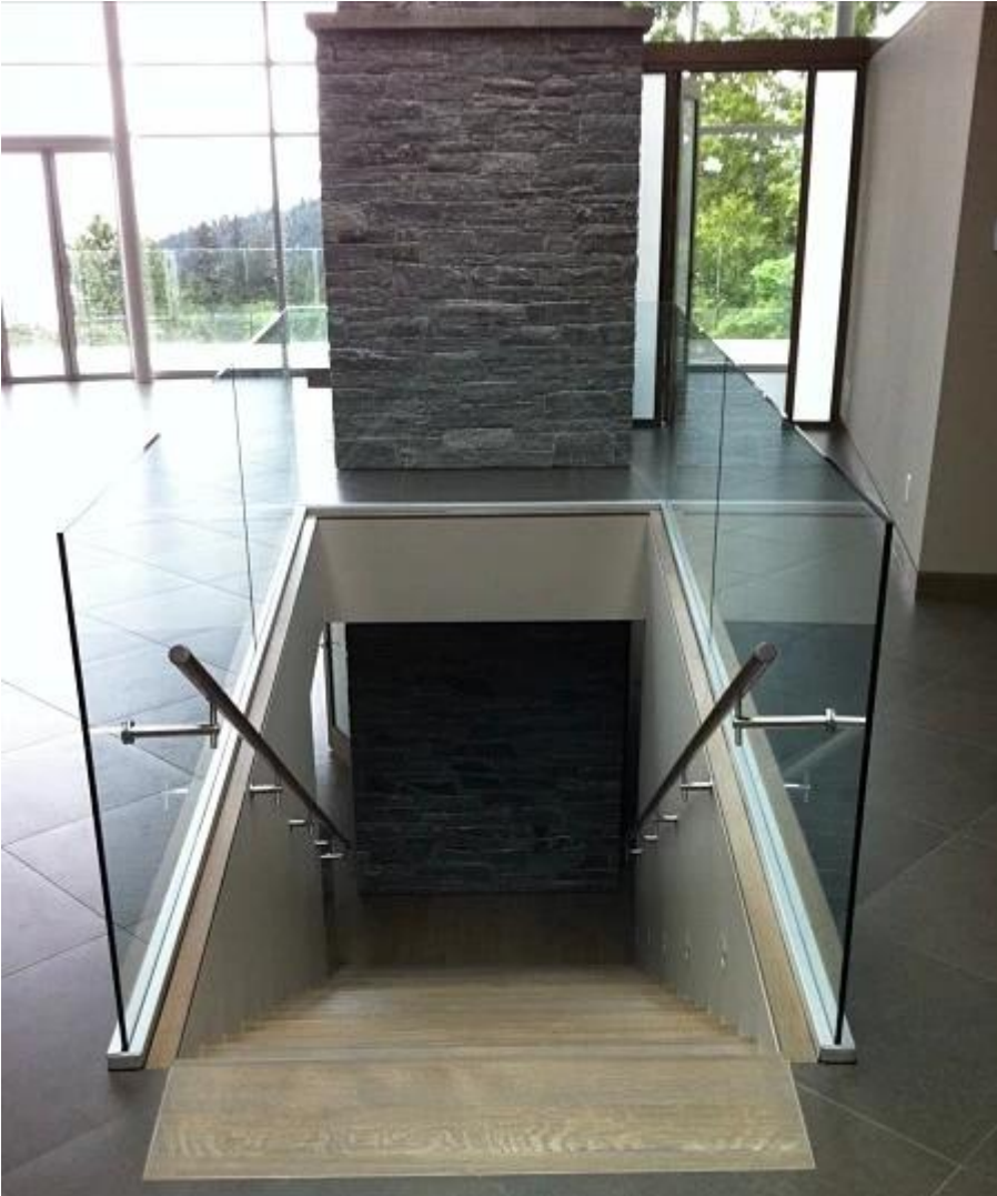
Installation photos for handrail bracket :
