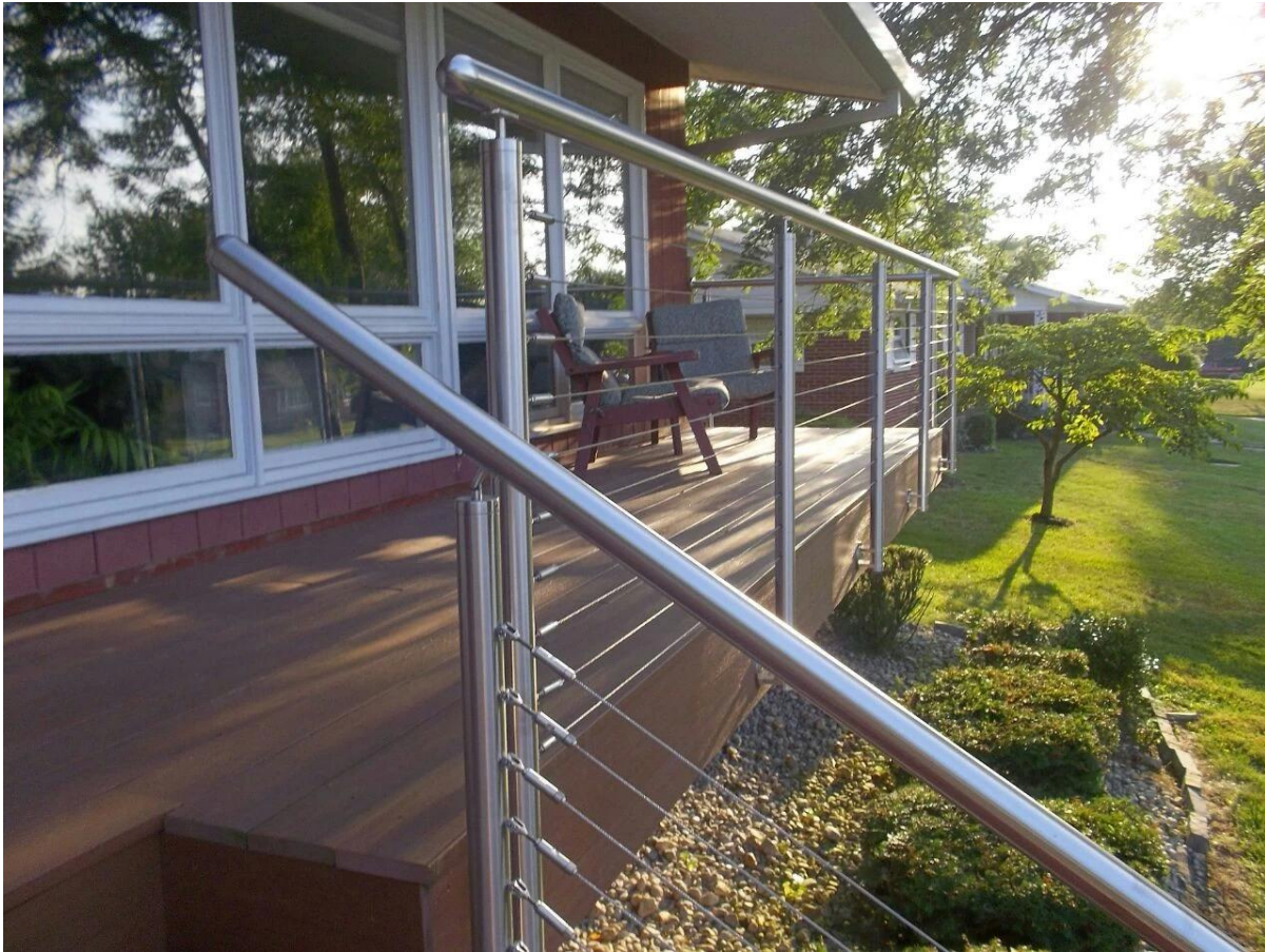
On stainless steel round post, diameter 50.8mm;
