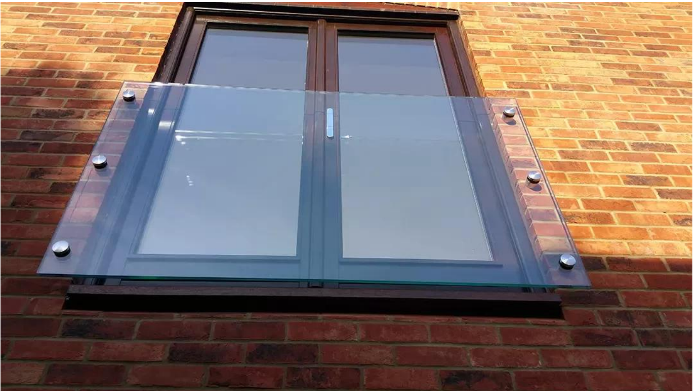
Installation photos of glass standoff railings-
