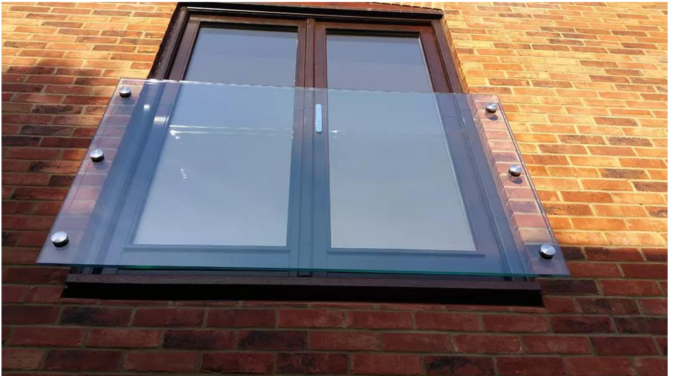
Installation photos of glass standoff railings-
