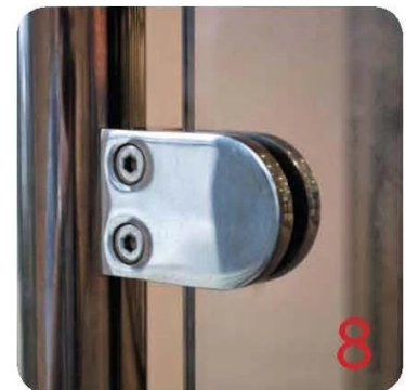
8 Tighten glass clamps with hex key, and check glass panel are secure with no movement.
