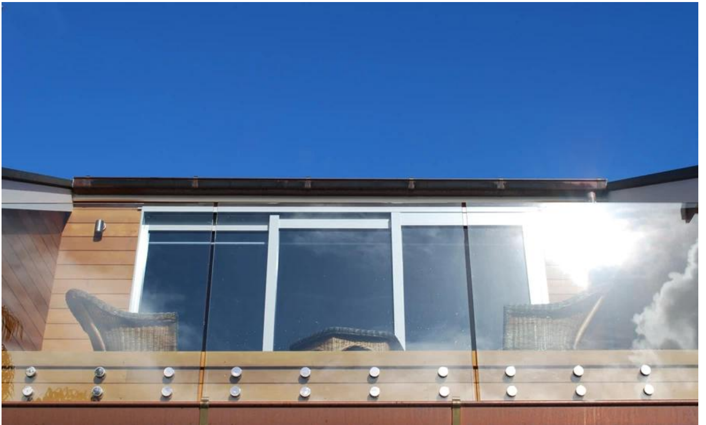
Installation photos of glass standoff railings-
