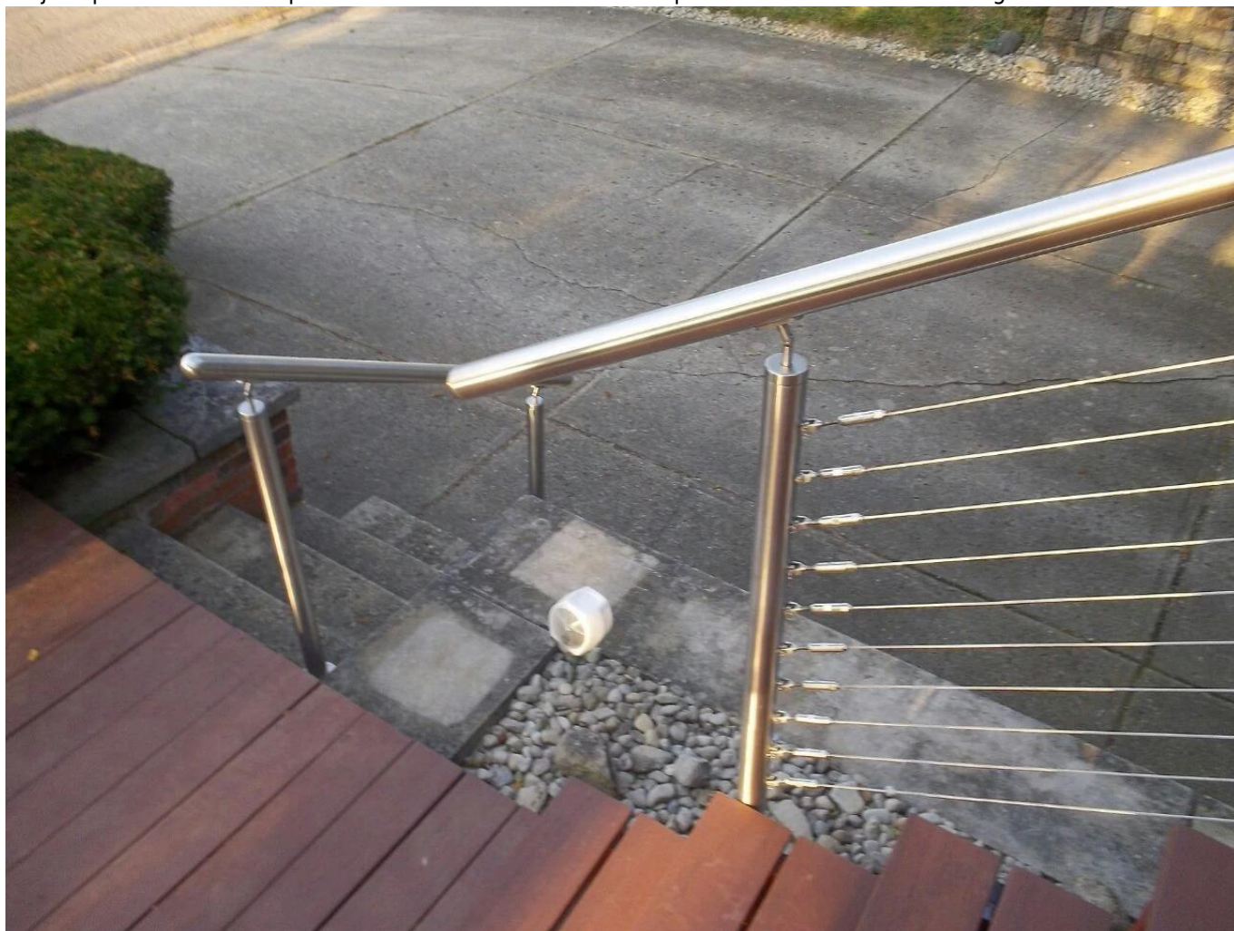
Project photos of wire rope balustrades with T803 Wire rope Threaded Turnbuckle Swageless-
