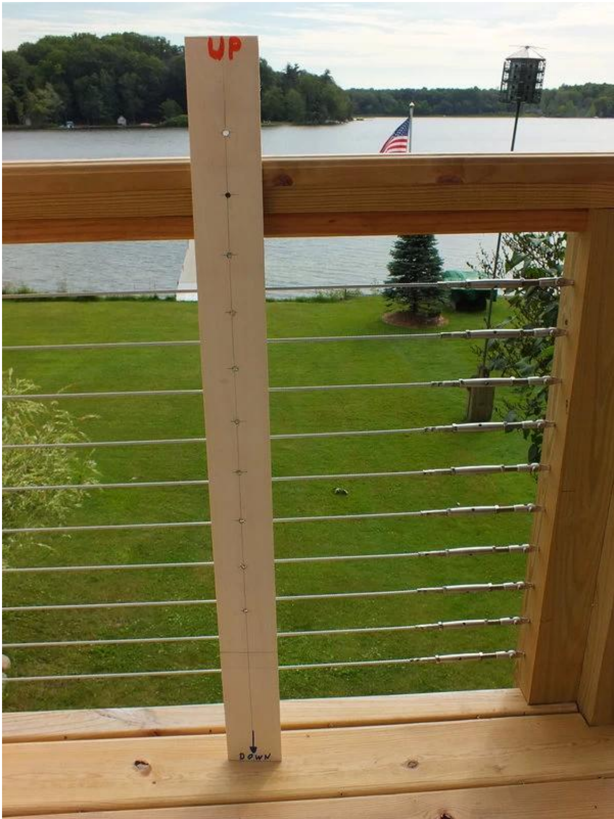
For staircase part
