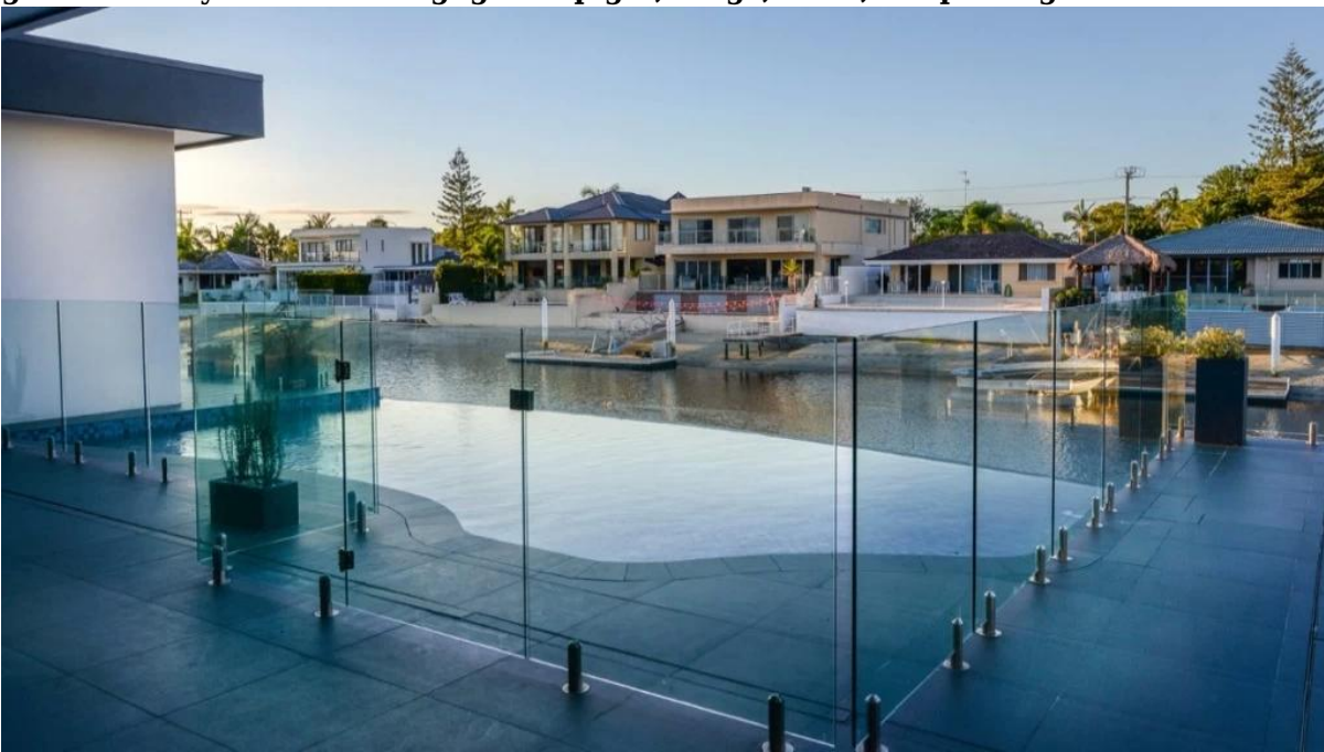
glass fence system including: glass spigot, hinge, latch, tempered glass
