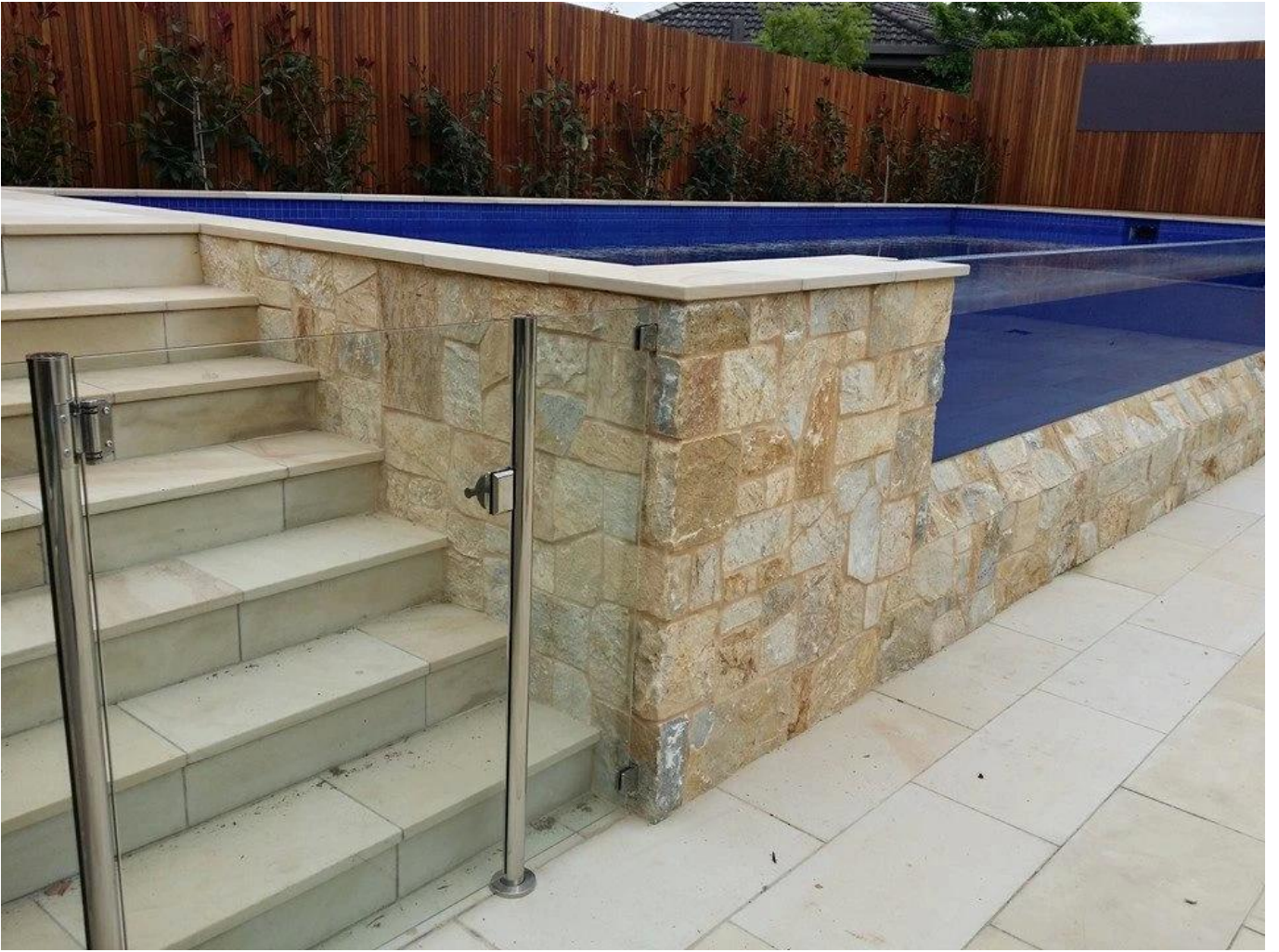
pool fencing spring loaded stainless steel 316 glass door hinge installed
