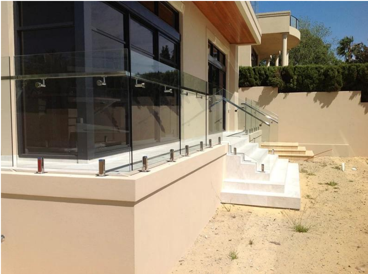
-Square spigot for balcony glass railing design
