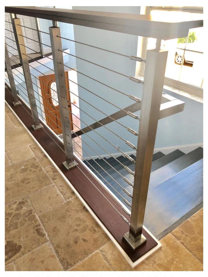
The Stainless Cable Railing Kit combines all the products needed to order and build a simple 38" residential height cable railing system with 3-10 posts. 42" or 46" commercial height available upon request.
