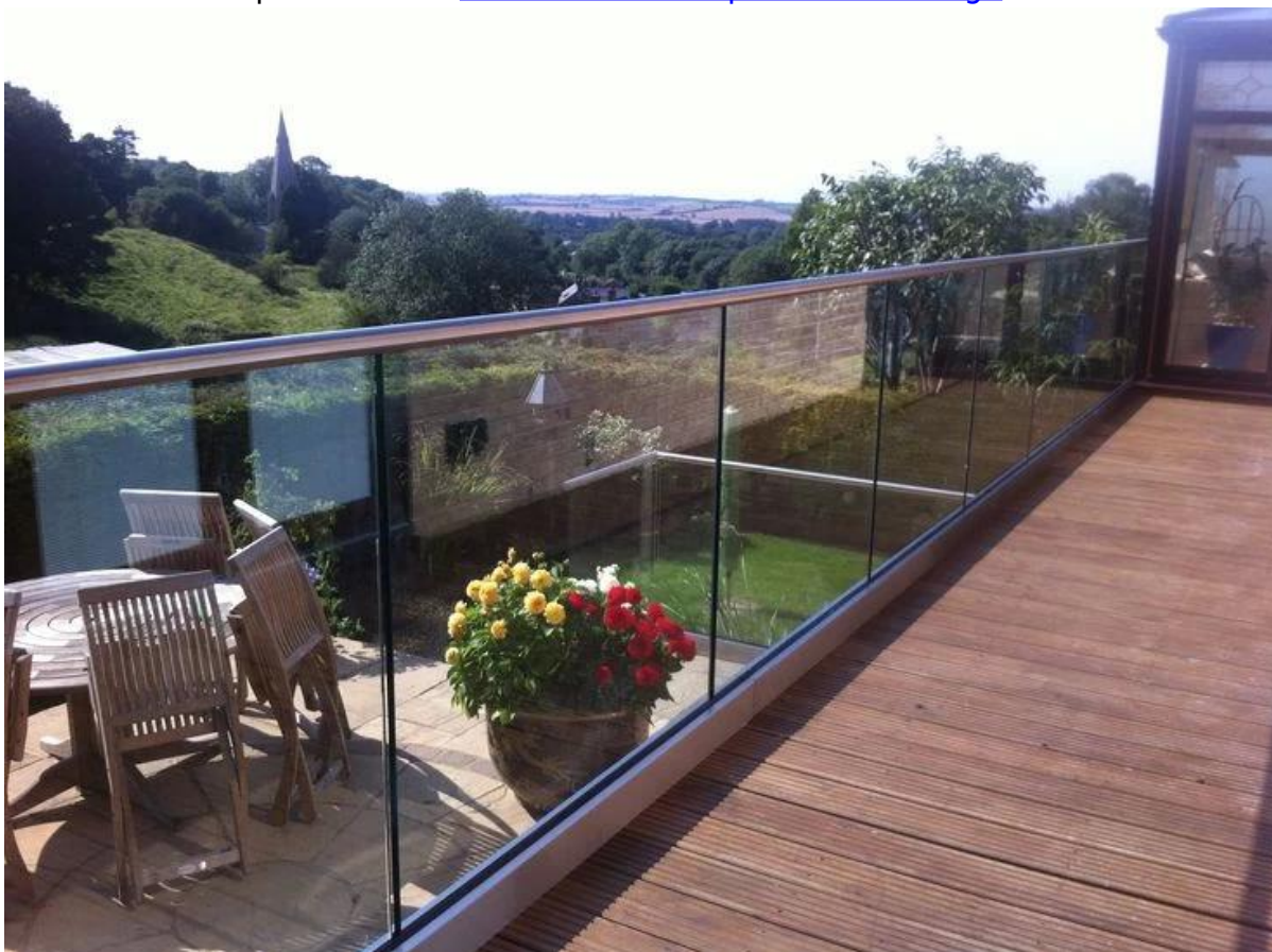
Project aluminum U-shape channel + stainless steel top handrail design
