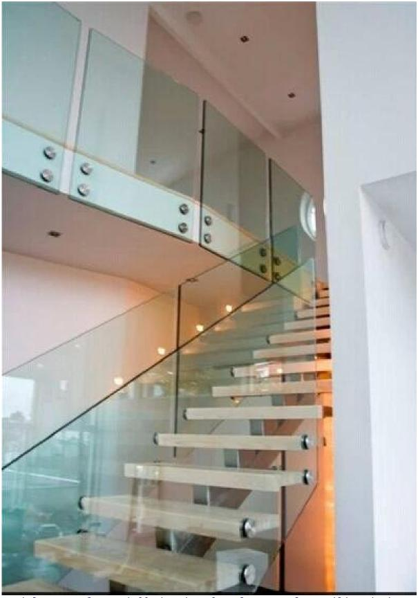
stainless steel standoff, bracket for glass panels, railing design
