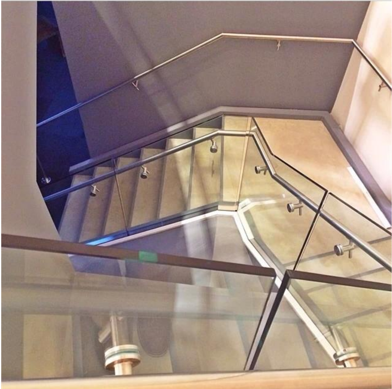
wall mount, stainless steel handrail brackets, suit for round tubing or pipe handrail
