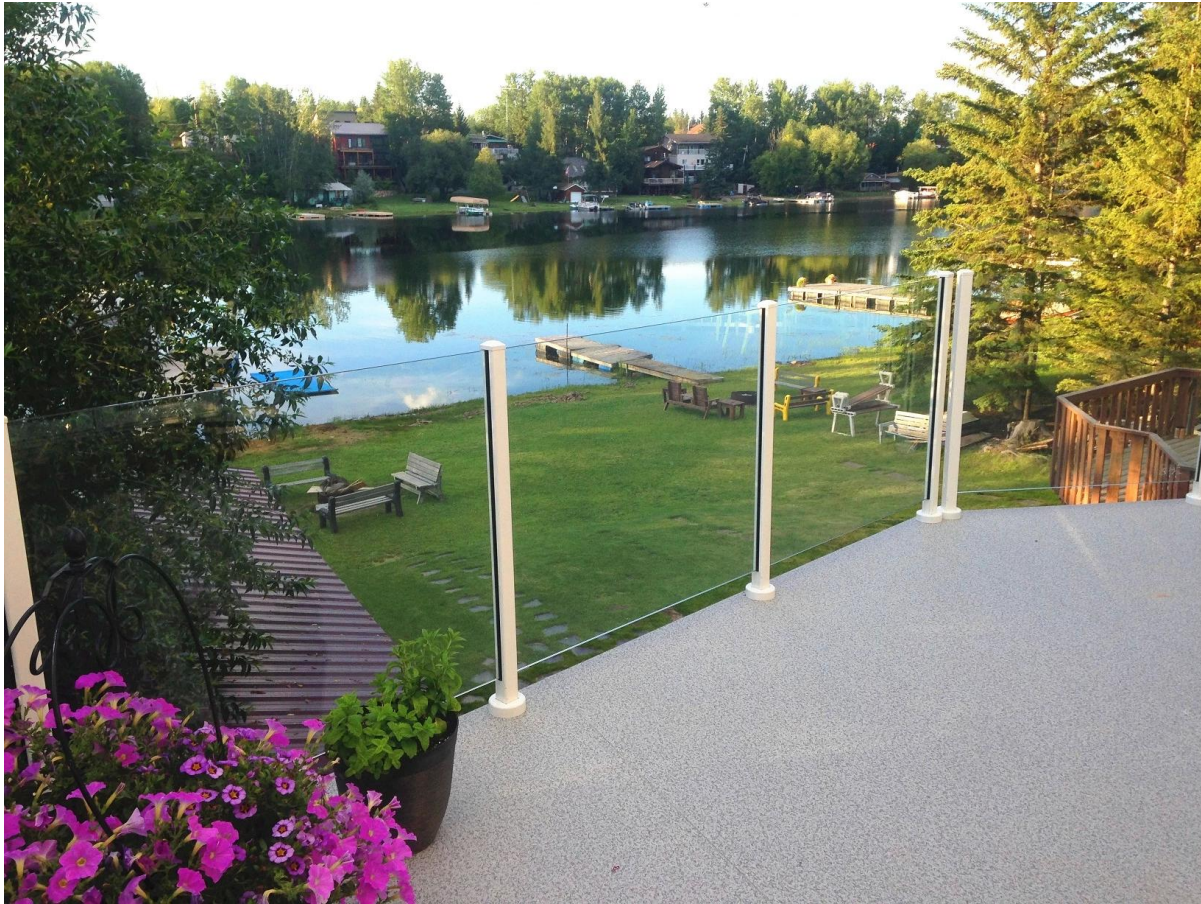
2) Round semi frameless glass fencing aluminum post : diameter 50mm x 3mm
