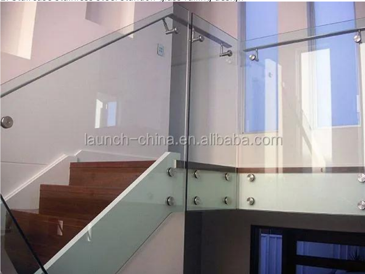
2. Staircase stainless steel standoff glass railing design
