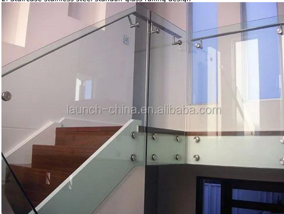
2. Staircase stainless steel standoff glass railing design
