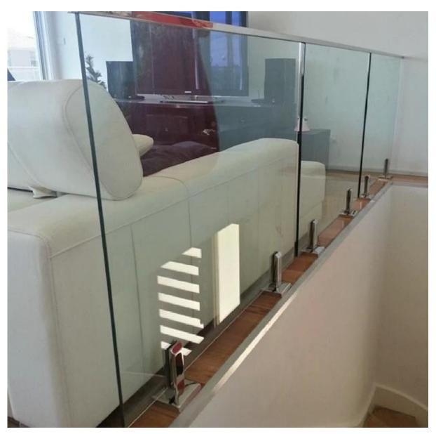
4. china supplier square stainless steel handrail fittings for 8-13.52mm glass railing package:
