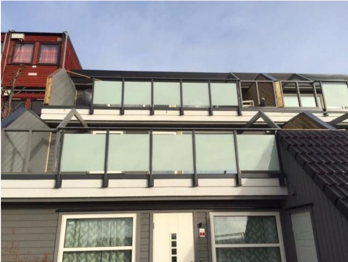
4. Aluminum profile handrail and rail packing photo , Aluminum post ,
