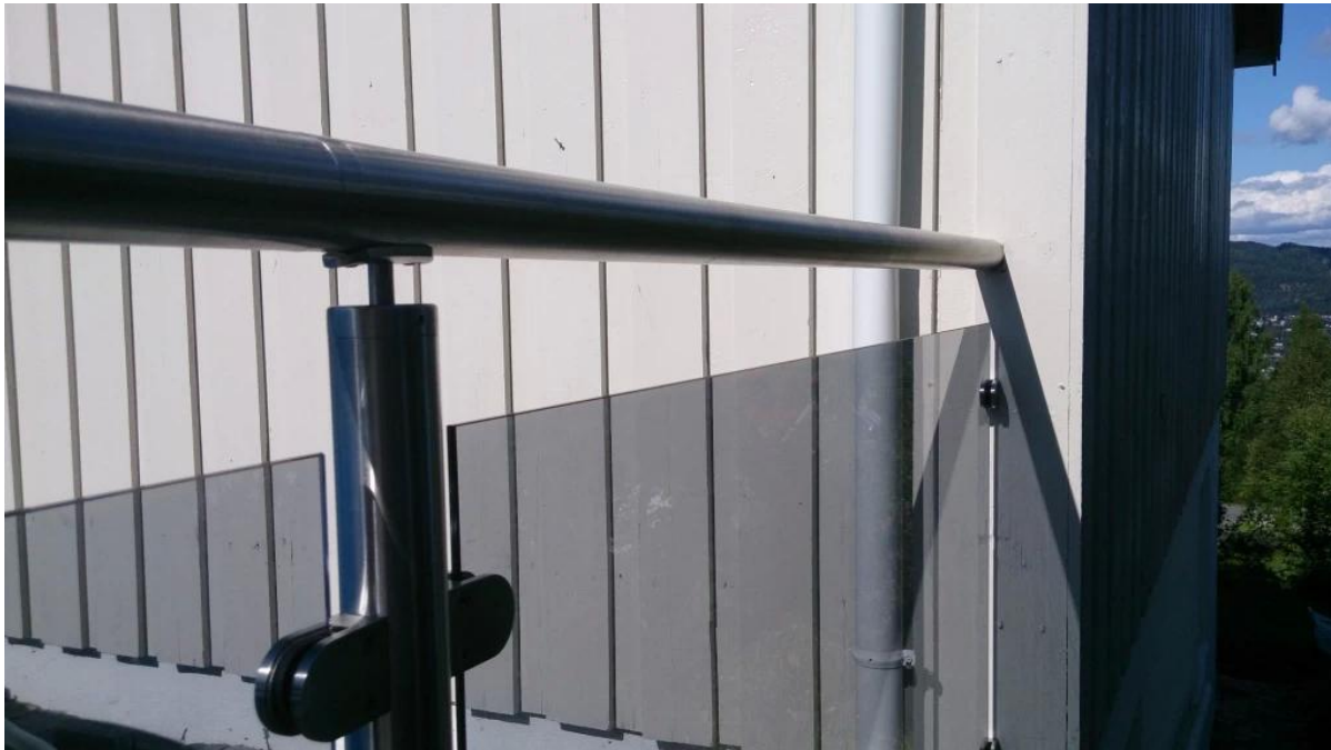
project show with handrail tube handrail size: dia 50.8mm
