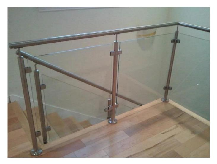
square glass balustrade post post size: 40\*40mm or 50\*50mm handrail size: 50\*25mm or 50\*50mm standard height: 1100mm, or as per your requirement
