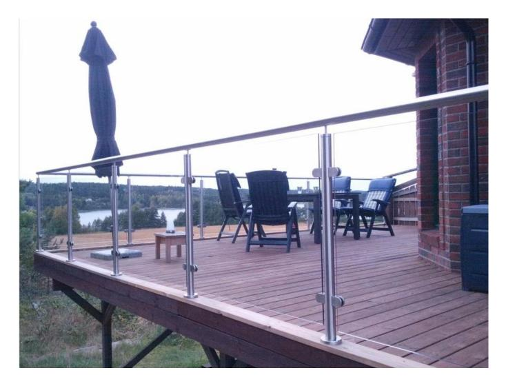
round glass balustrade post post size: dia 43mm or 50.8mm handrail size: dia 43mm or 50.8mm standard height: 1100mm, or as per your requirement
