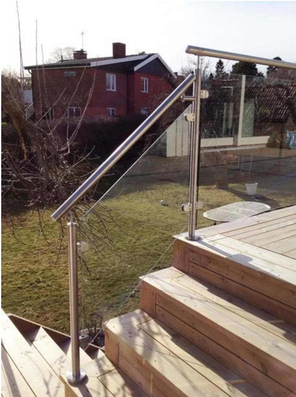
glass balustrade post railing for stairs
