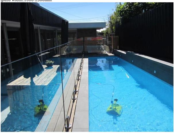
glass balustrade system, frameless glass balustrade system, framless glass balustrade with stainless steel spigots and tempered glass
