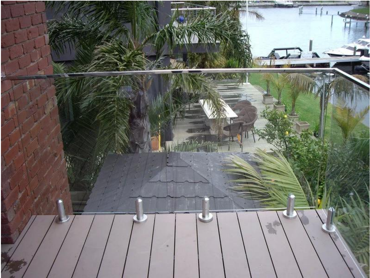
Outdoor deck glass railing
