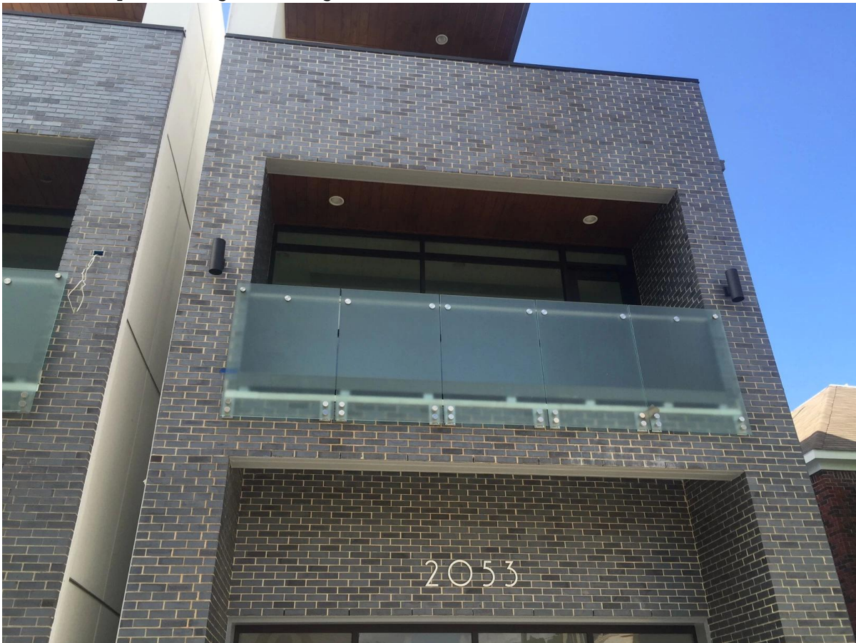
Installation photos of glass railing standoff bracket
