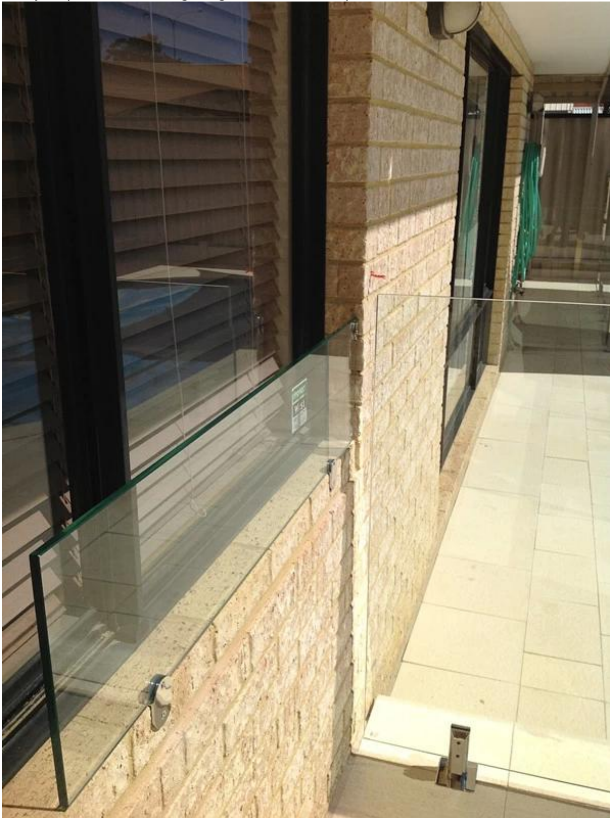
- Project photo of 180 degree glass to wall clamp
