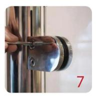
Fit glass panel into position, install second half of glass clamp secure with provided hex screws.
