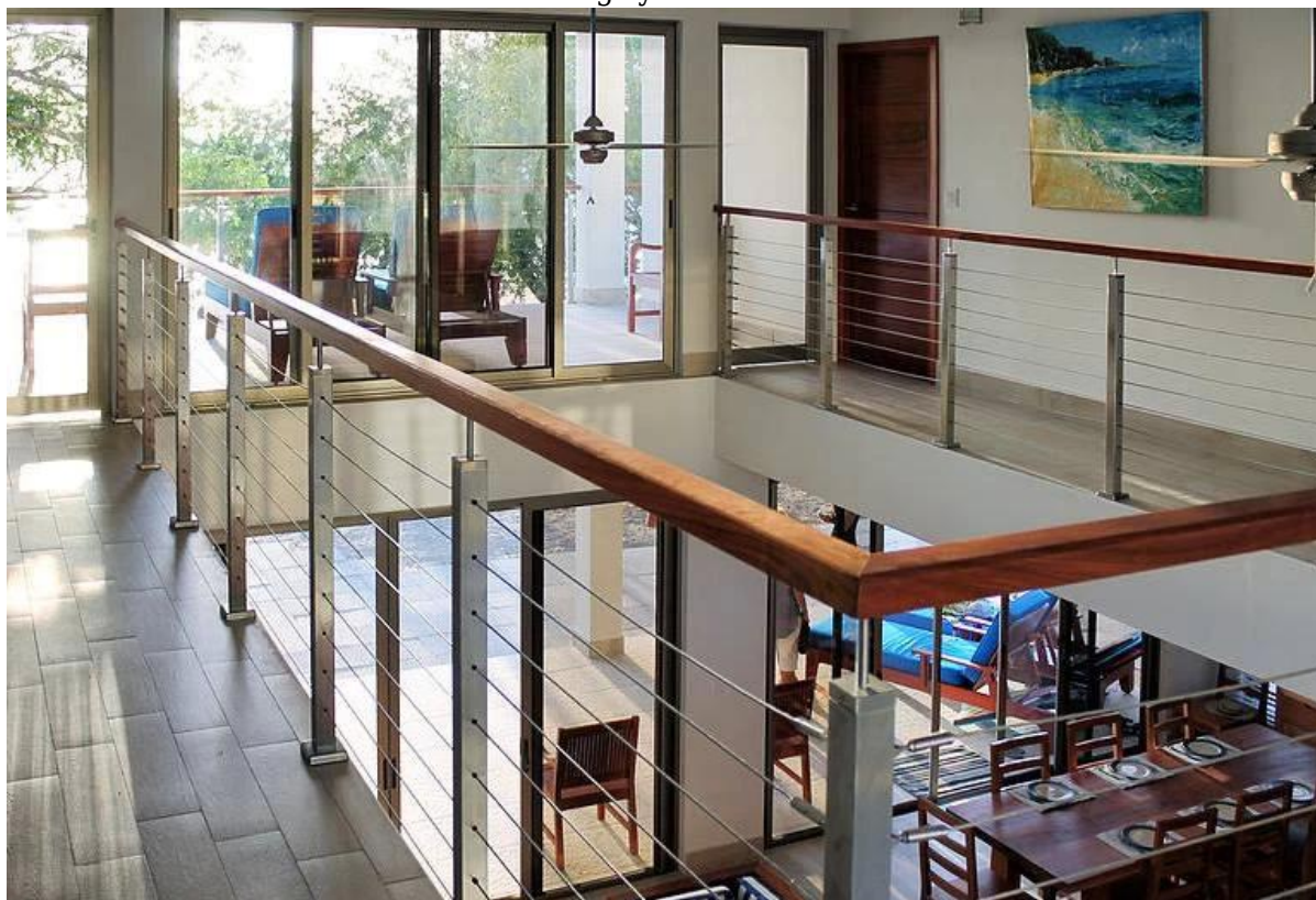
stainless steel 316 staircase cable railing systems
