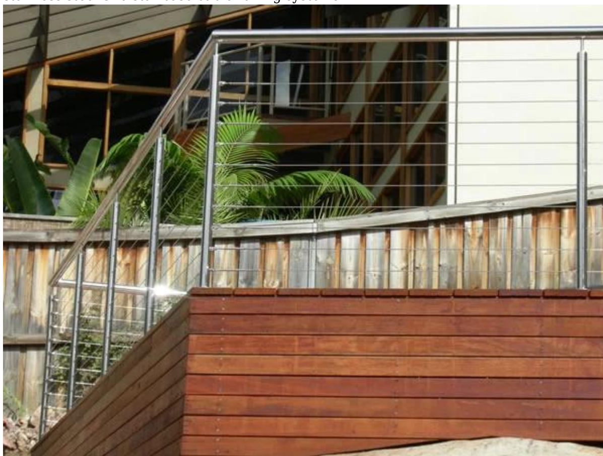
stainless steel 316 staircase cable railing systems
