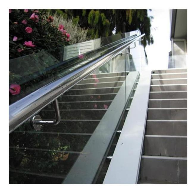
Model No.: P708 material: stainless steel 304/316 finish: satin or mirror polished for tube size: dia 42mm or 50.8mm
