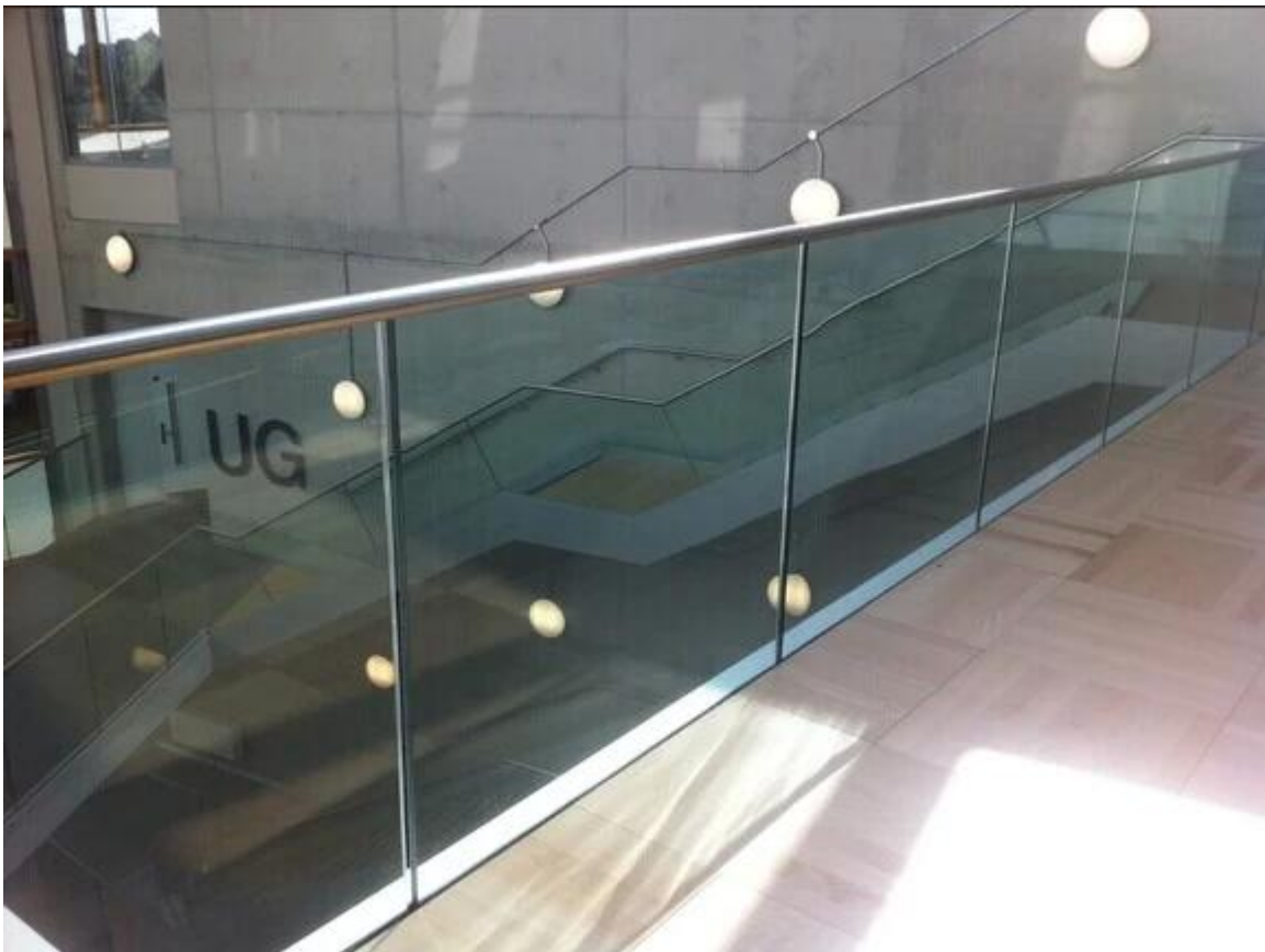
Square top rail material: stainless steel 316/316L
