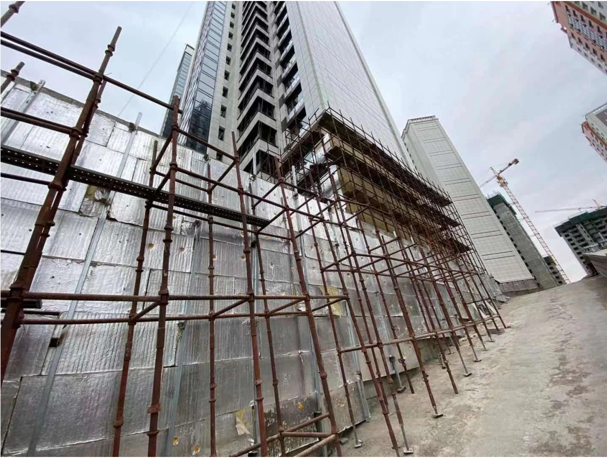
Production of slot balustrade handrails & glass panels-
