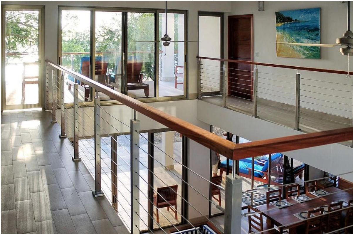
Installation photos of stainless steel cable railings , top can be wood handrail .
