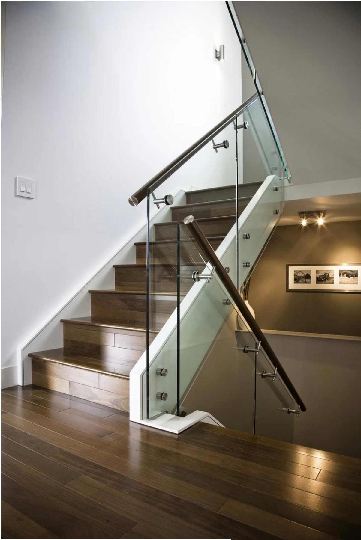
Fixed stainless steel handrail brackets project :
