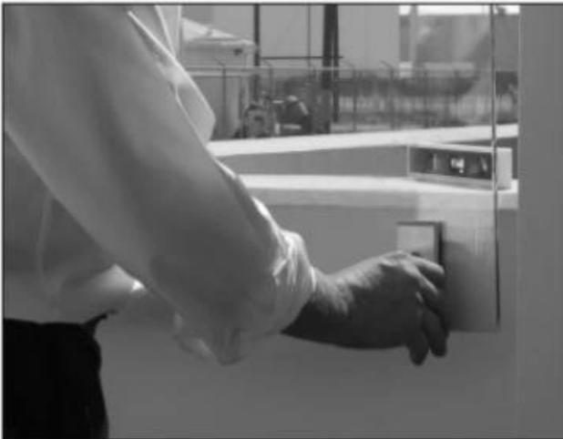
Place the gaskets against the base fitting, both back and bottom lip, then set the glass panel on the base fitting. Next place the front gasket against the glass panel along with the front plate and secure to the base fitting by tightening the two screws. Don't tighten all the way, leave enough play to adjust the glass panel.
