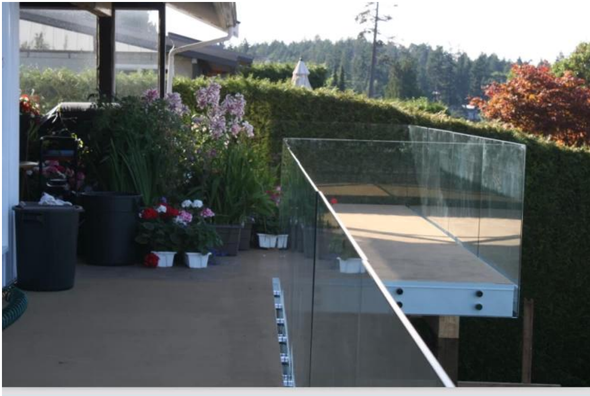
Installation of glass standoff with mounting plate on staircase
