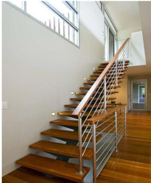
单龙骨楼梯 Single Stringer stairs 不锈钢拉杆木扶手 Stainless steel rod wooden handrail
