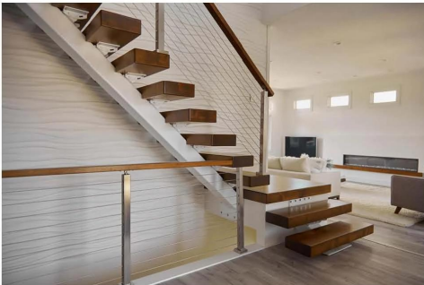
单龙骨楼梯 Single Stringer stairs 不锈钢拉杆木扶手 Stainless steel rod wooden handrail
