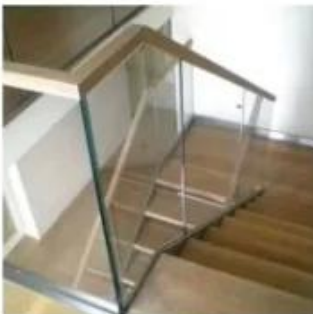
U channel glass railing
