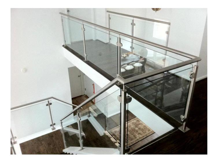
square post post size: 40\*40mm or 50\*50mm handrail size: 50\*25mm or 50\*50mm
